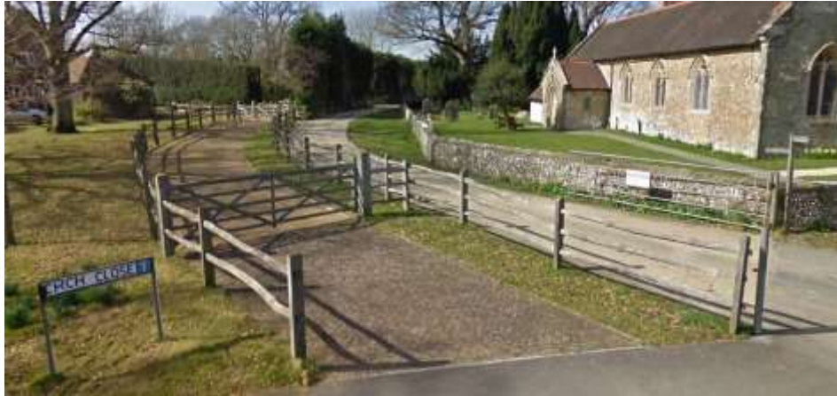
Existing access routes (Google StreetView)
